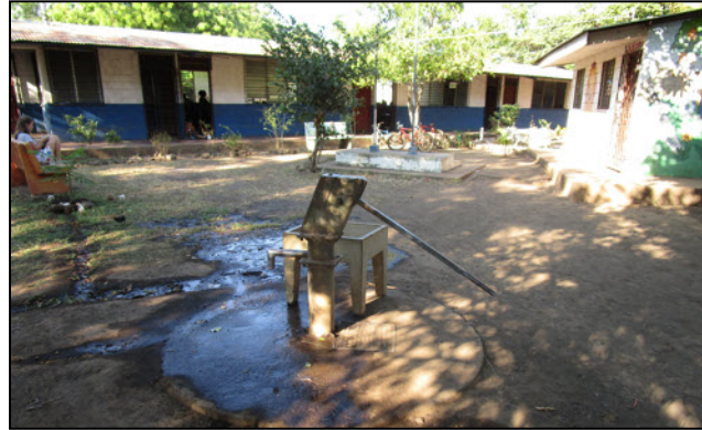
The community of Nueva Vida in Goyena has five deep wells that provide clean water for the community, like this one at the school. Many families have hand dug wells which now need to be regularly deepened as the water table falls.
